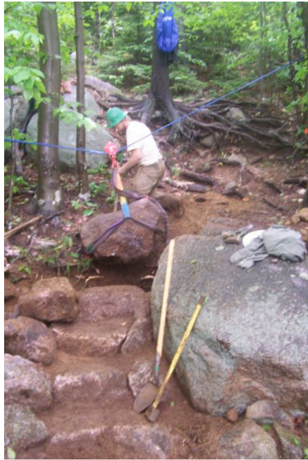
Photos 3 and 4: Step stones being set off a skyline
