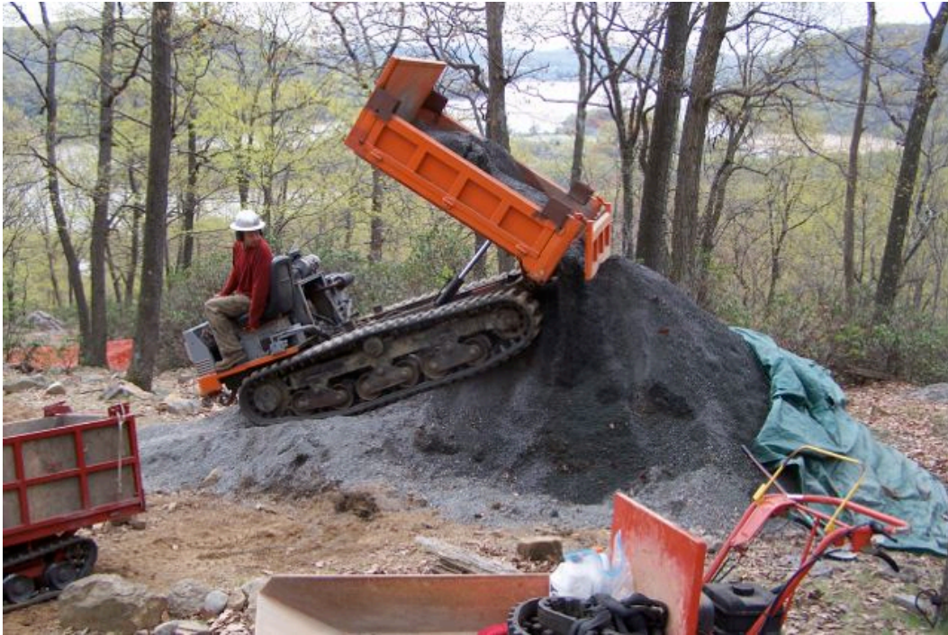
Photo #1: 60" wide tracked carrier moving aggregate
