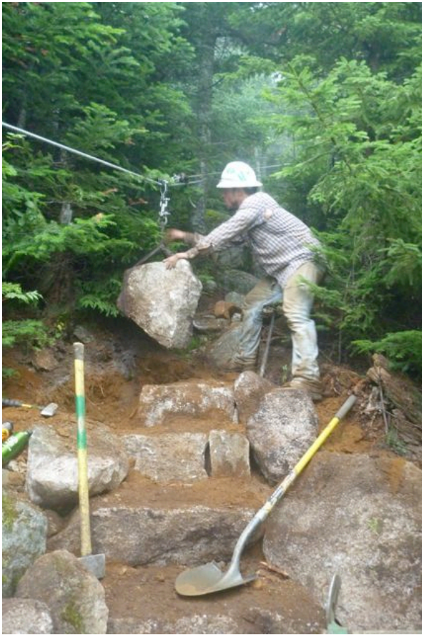
Photos 3 and 4: Step stones being set off a skyline
